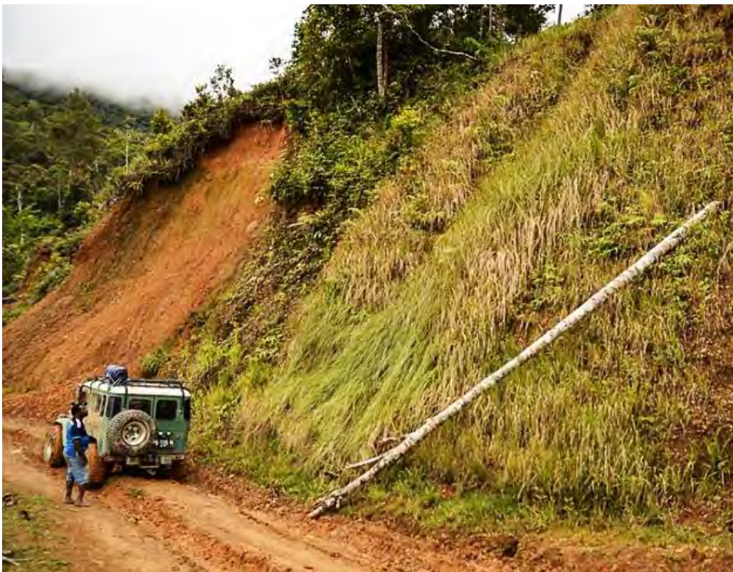
Figure 16. Success! Twelve (12) months after planting, the control on the left portion of the slope continues to experience erosion while on the right-hand side the Vetiver is protecting the slope.
