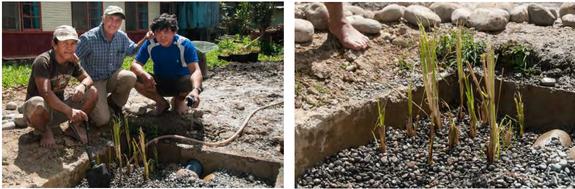
Figure 4. Small HSSF Wetland in Wamena at end of construction.
