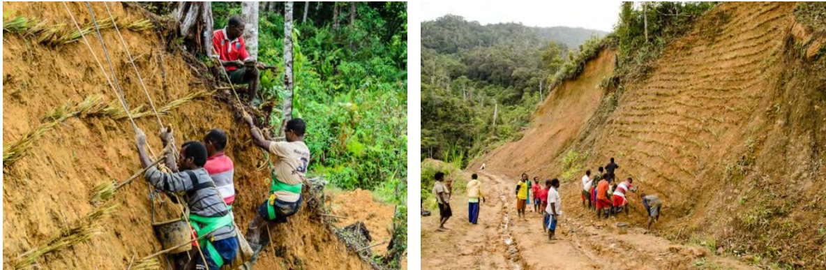
Figure 15. Left: Using rappelling equipment to plant. The slope varied from 60° to almost 90° in some sections. Right: Nearly finished planting.
