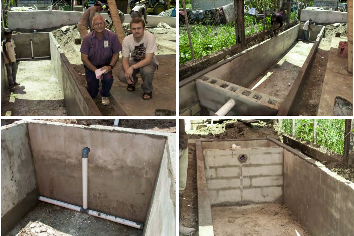
Figure 2. YAJASI's HSSF Wetland in construction. Top left: YAJASI technicians responsible for implementing the design. Top right: The wetland. Bottom left: Design of the intake system. Bottom right: Looking towards the outflow system and vertical leach chamber. Note the underlying brick construction can be clearly seen in this photo.
