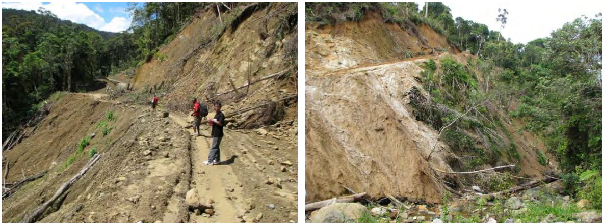
Figure 12. Left: Surveying the road. Right: A typical landslide.
