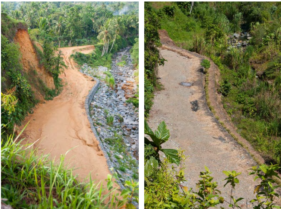
Figure 7. (Left) Following first gabion installation and before planting with vetiver, October 2009 and (right) following planting and trimming, December 2012.
